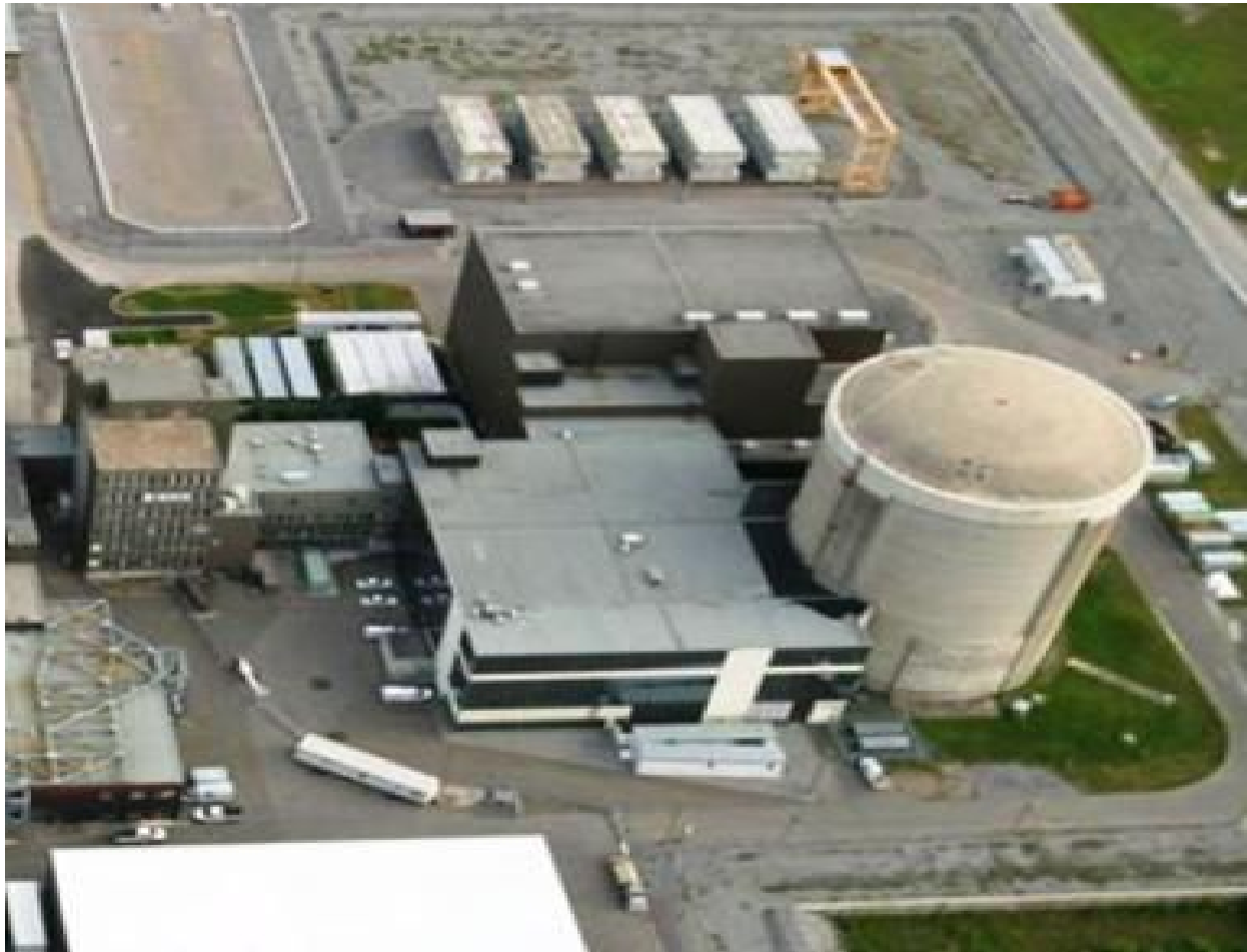
Figure 2: Gentilly-1 Prototype Reactor in Bécancour, Québec
