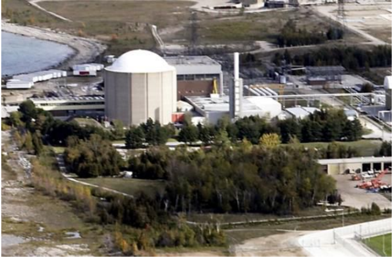
Figure 1: Douglas Point Prototype Reactor in Tiverton, Ontario
